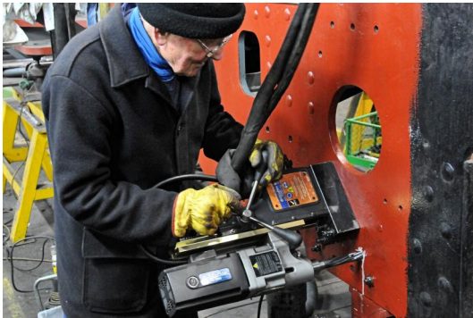
Reaming holes for fitted bolts
