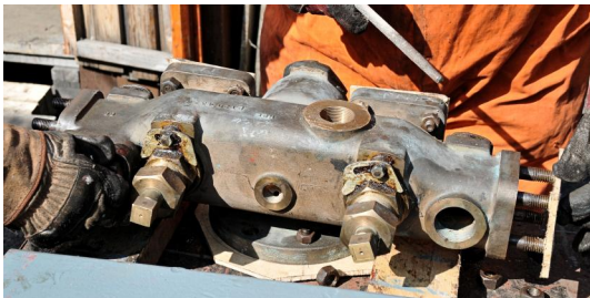
Fitting covers to the main steam manifold
