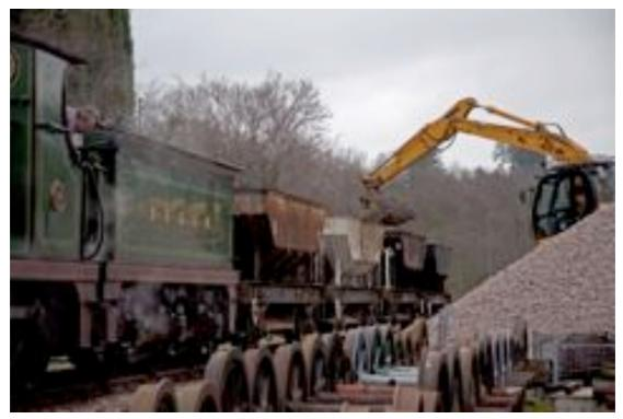
The 27<sup>th</sup> started cloudy but brightened up, and we headed up to between Vaux End and Black Hut to tackle some of the worst dipped joints. These needed jacking and packing. Keeping our generators on board the Wickham to ease the task of moving locations we see a close-up of proceedings. Here we see Jon with the cant stick (in effect a long spirit level) and Julian about to operate the track jack, raising the track as directed by Jon.
