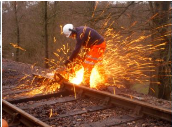
Wednesday evening. Final cutting in of the closure rails as it gets dark.
