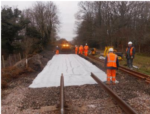
End of Thursday afternoon. Rails out and terram down after only half a day.
