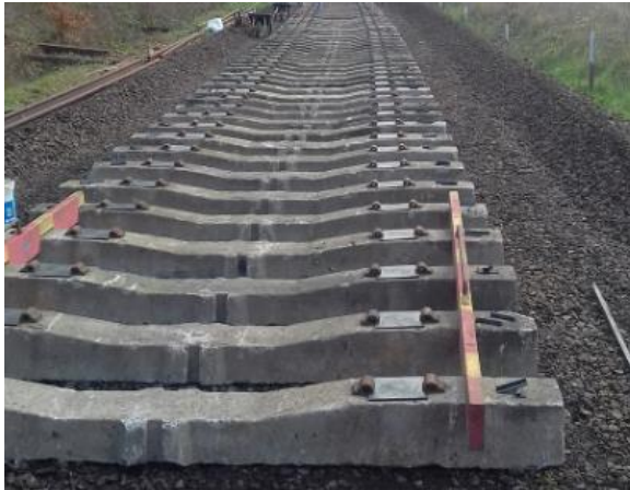
Sleepers aligned ready for the rail. Photo: Bruce Healey.
