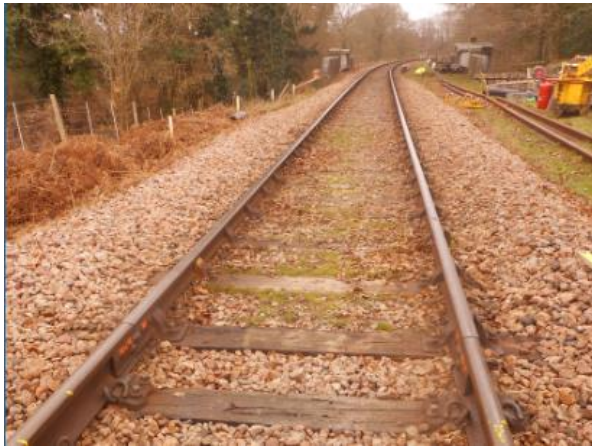
The first panel to be changed, 50 yards before Sloop Bridge.
