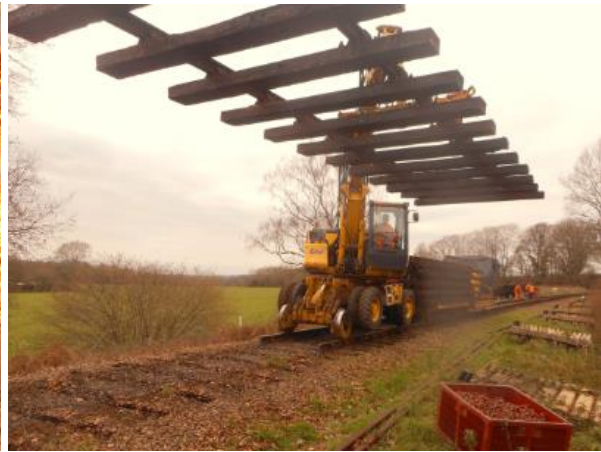
Lifting out the half panels
