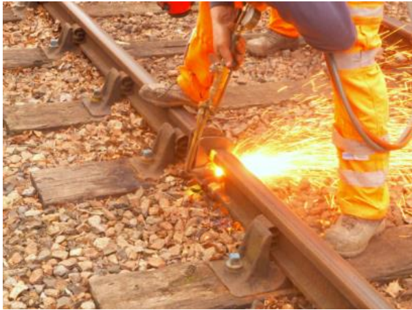
Gas cutting the rails
