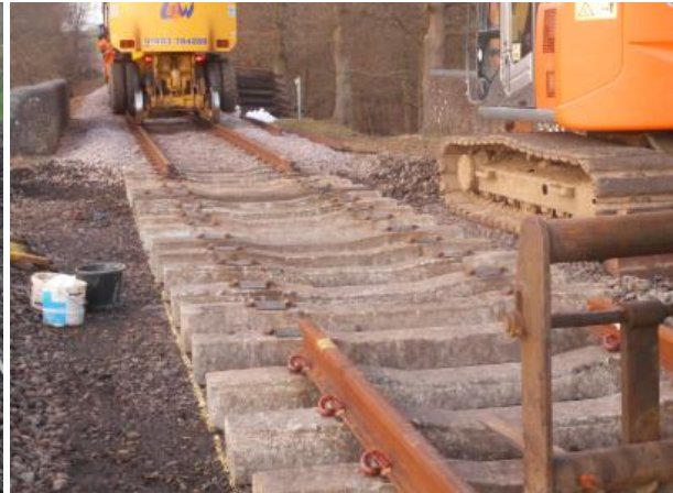
Less than 30 feet to go. Sleeper position marks can be seen on the rail head.
