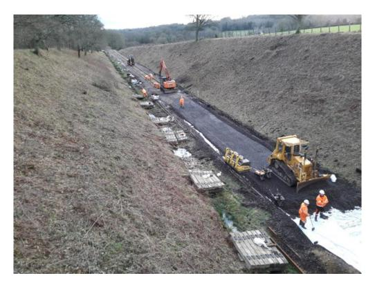
Finally, two pictures show how we left it at the end of Friday, one from the top of the bridge just before we stopped putting out sleepers and one looking back along the line from under the bridge. The straightness was due to the use of our new (gifted) theodolite which we are very pleased with and the smoothness is due to the use of our laser with the laser bulldozer. This makes tamping a lot easier as is as good as main line standards.
