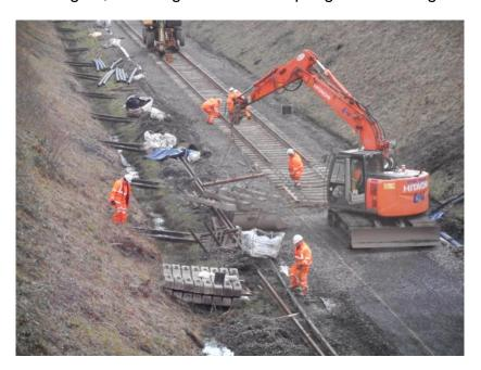
After bulldozing the ballast flat and compacting it smooth with the triple Wacker, the yellow line was painted on the ballast in line with the sleeper ends to help the team to place the sleepers accurately, as seen being craned in four at a time suspended from a lifting bar. These are placed with their centres on average 653.27mm apart!! But normally within 5mm of that giving 28 sleepers per panel instead of 24 as was the previous standard.
