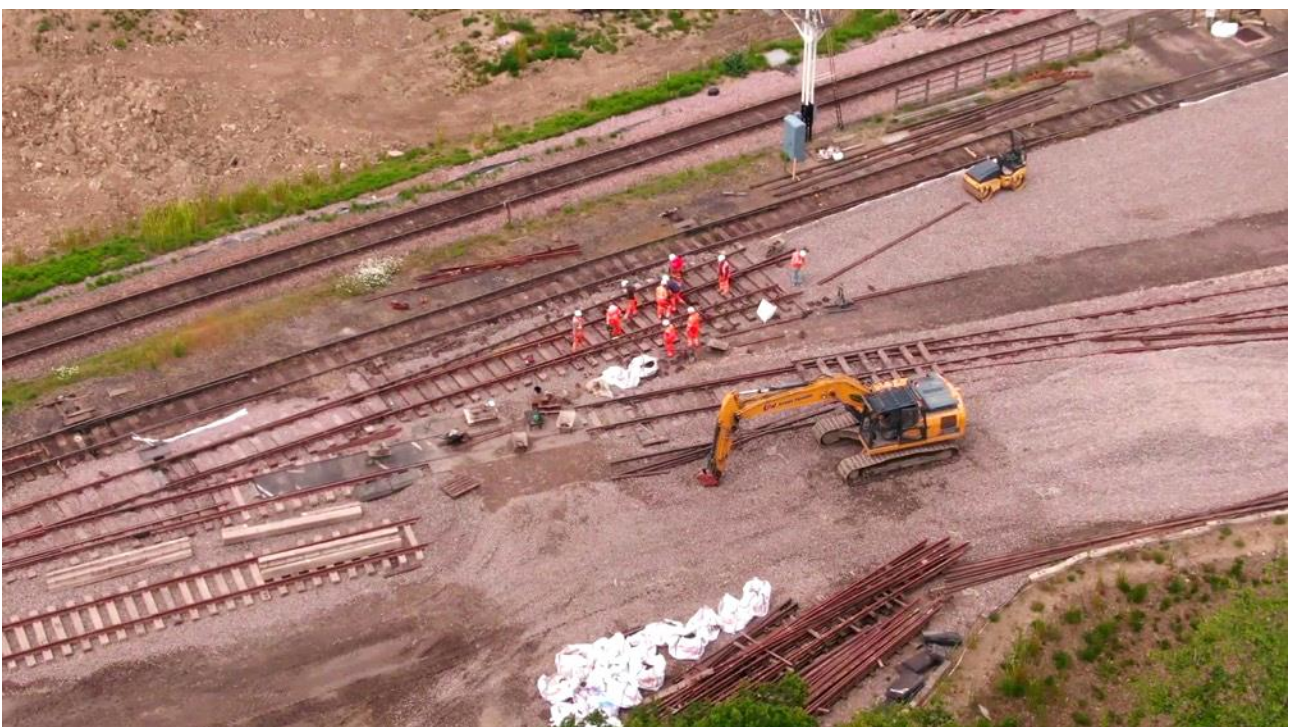
Working on the three way point (John Harwood)
