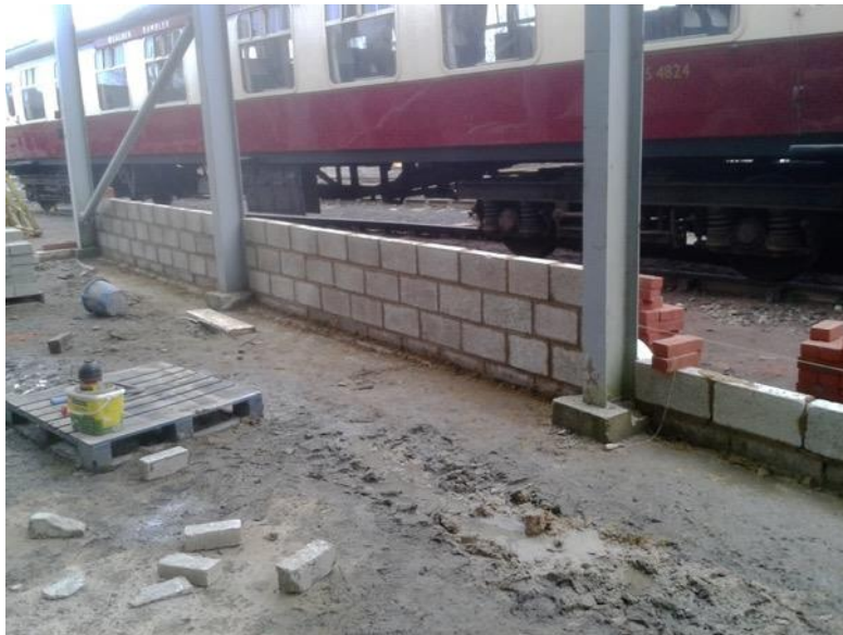
The interior blockwork of the dwarf wall on the western side of the maintenance road (Bruce Healey).
