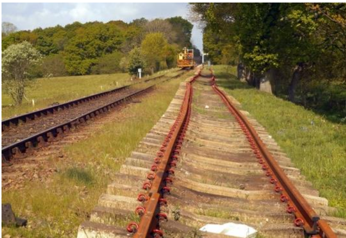
New panels placed beside the existing track.
