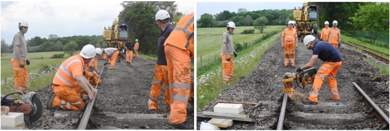
Measuring and cutting in the last panel.
