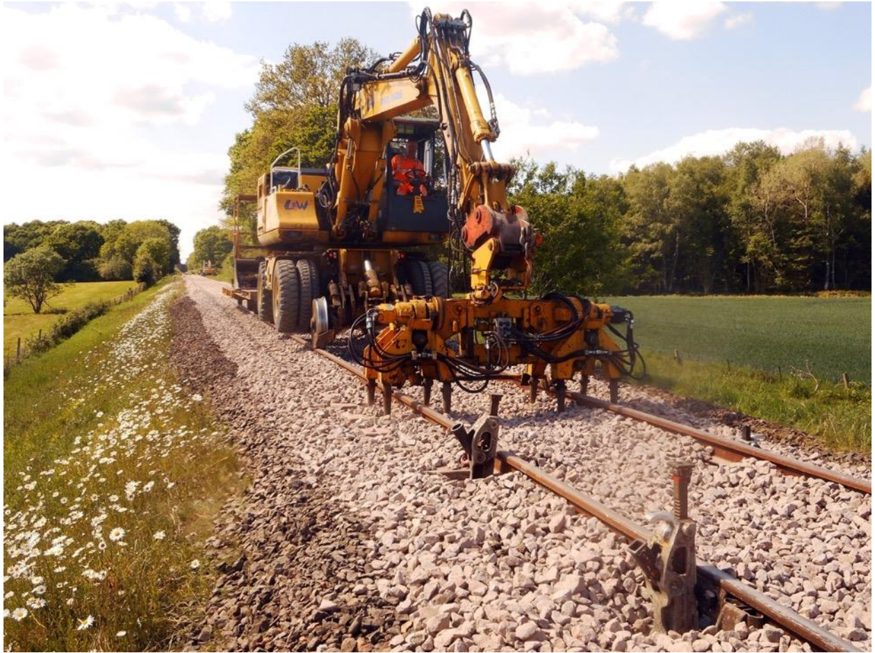
Tamping the ends of the job.
