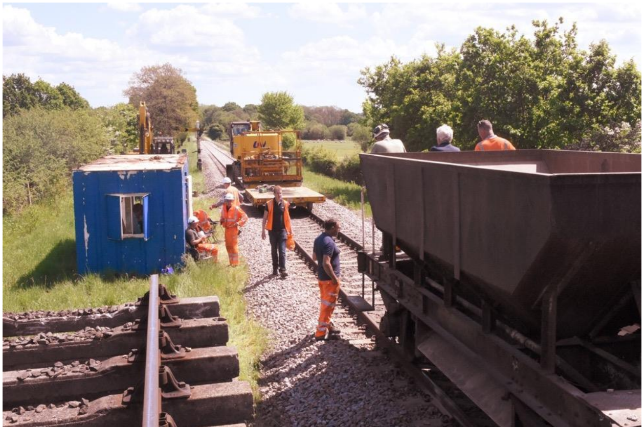
Standing back and admiring the finished job
