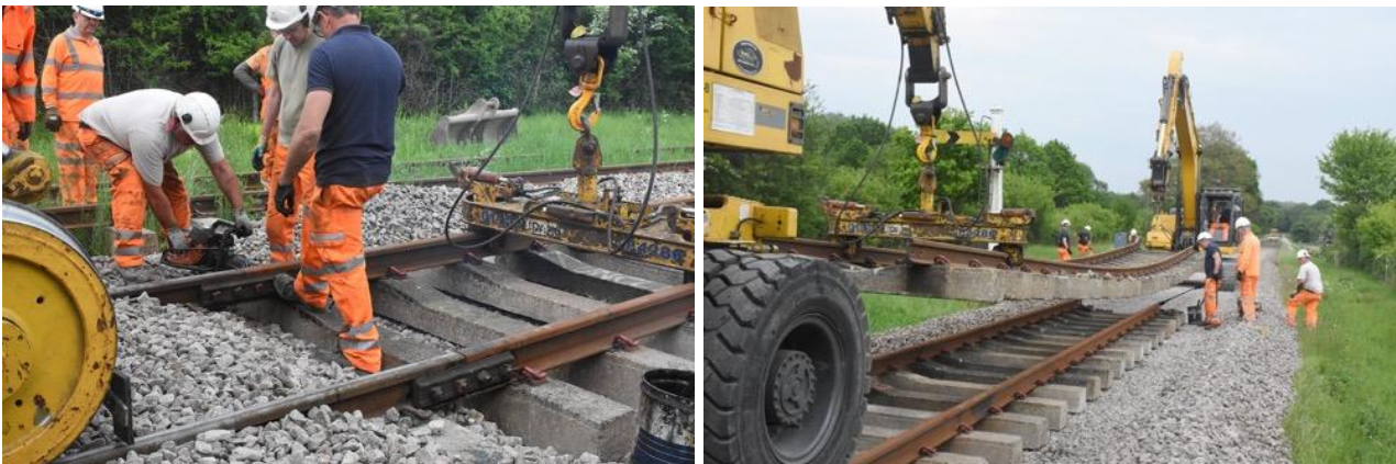
First panel being bolted in place.
