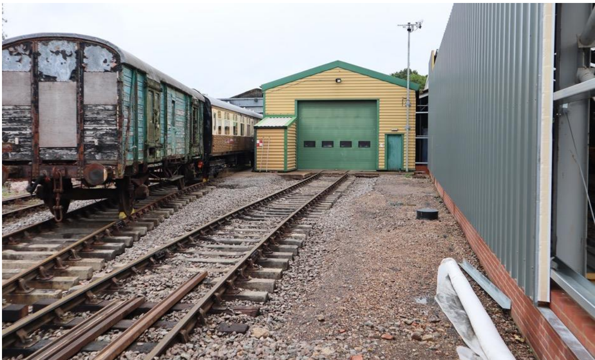
Track into D road (paint shop) and B road of the existing shed now completed
