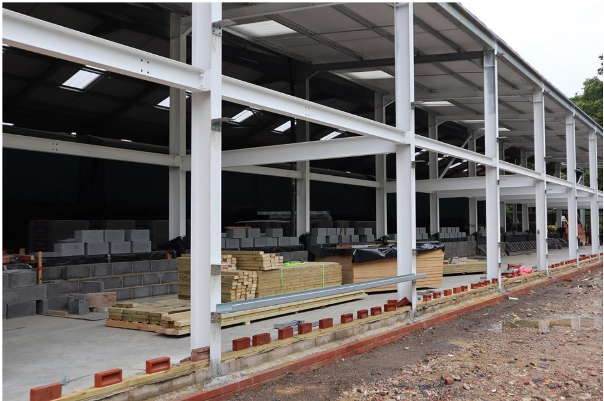
HSC steelwork cleaned, and painted with protective paint
