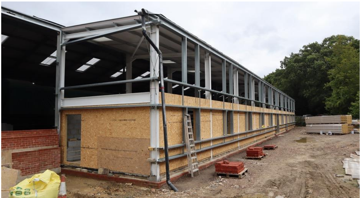
Completed ground-floor studwork
