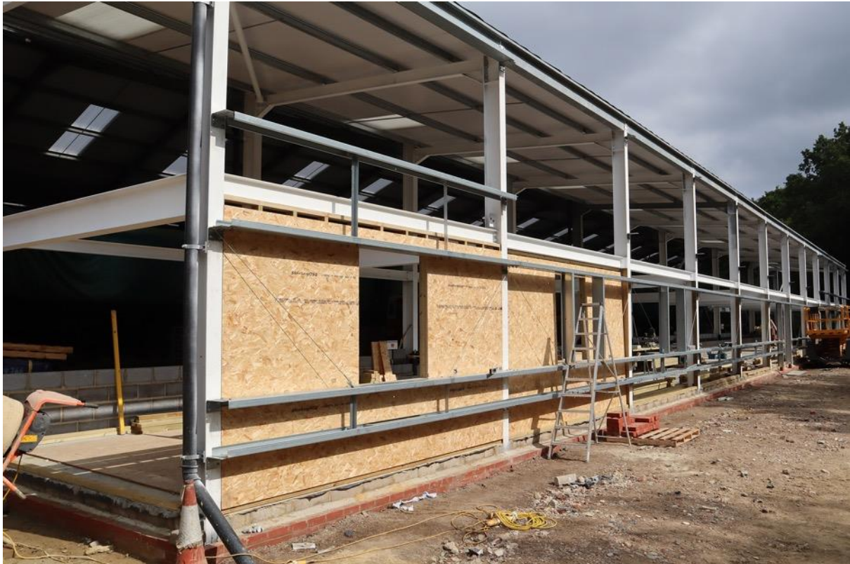
Fixing of cladding support rails in progress
