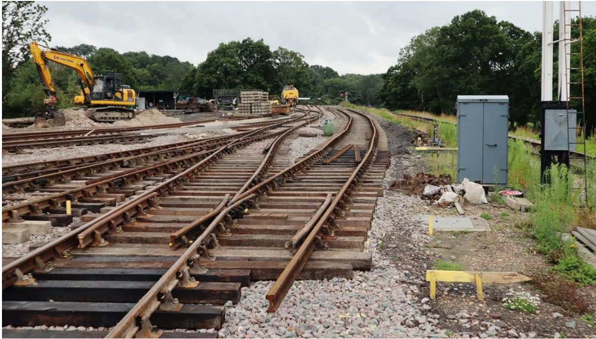
Crossing installed for new point
