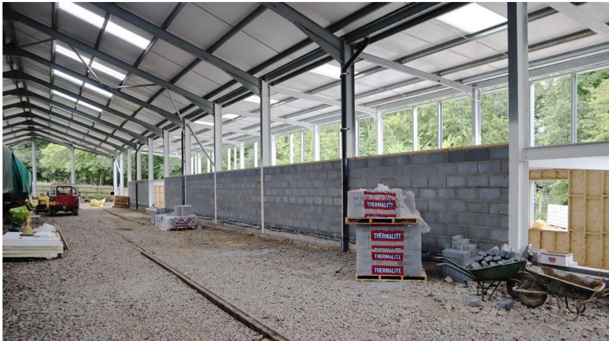
Blockwork on the ground-floor interior (shed) side of the HSC
