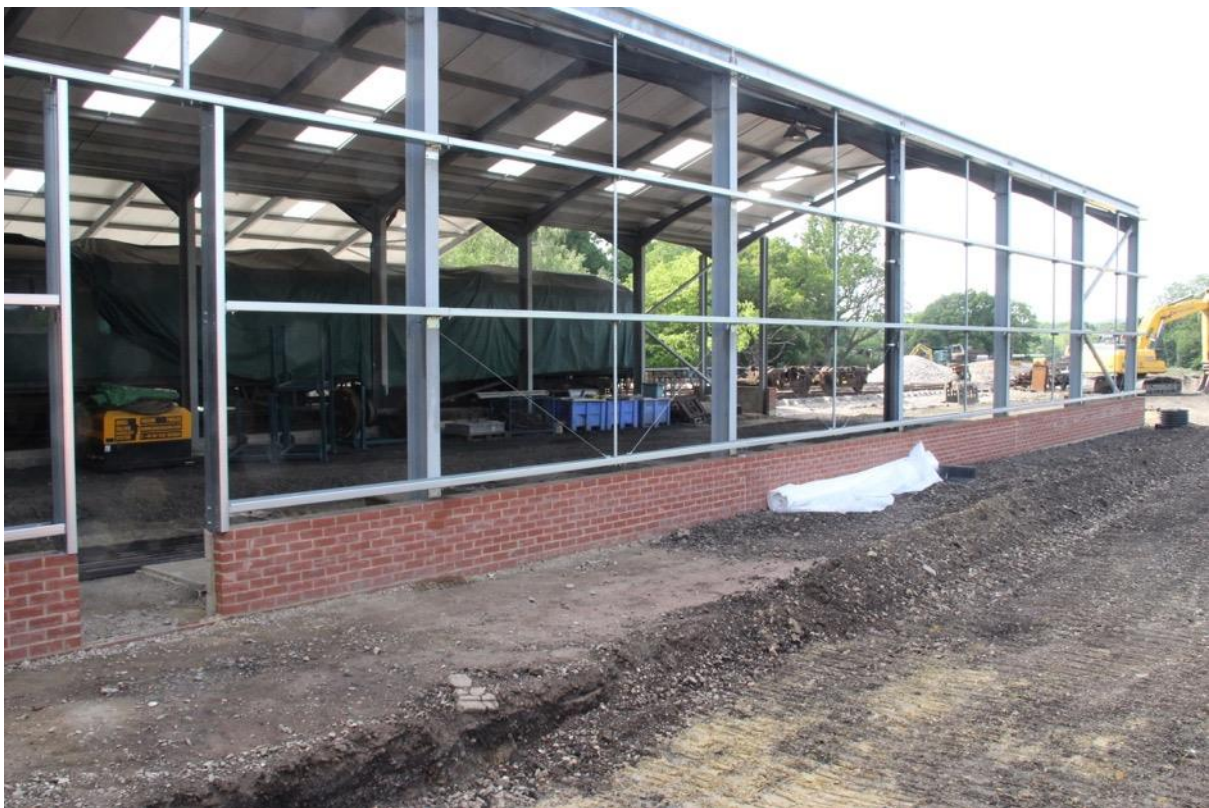
The western side (facing the railway) with the cladding rails complete
