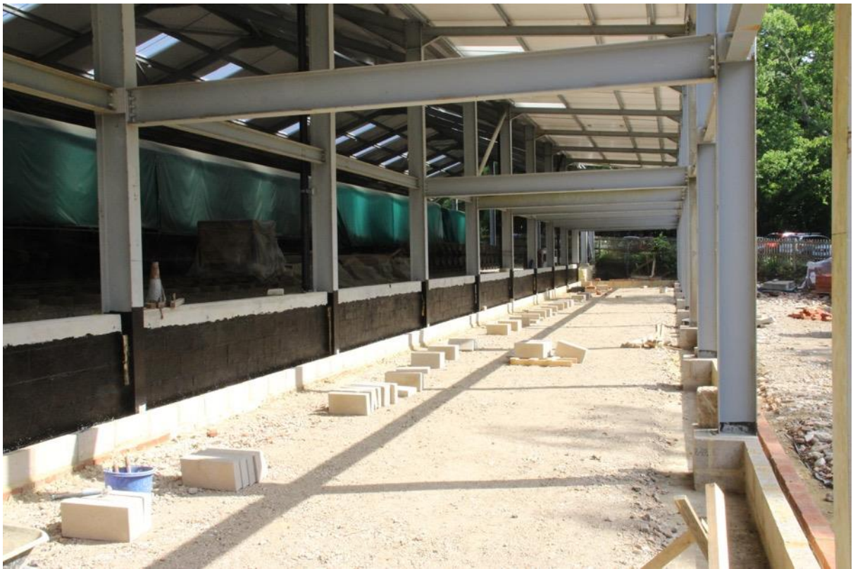
The HSC ground floor being prepared for the concrete floor slab
