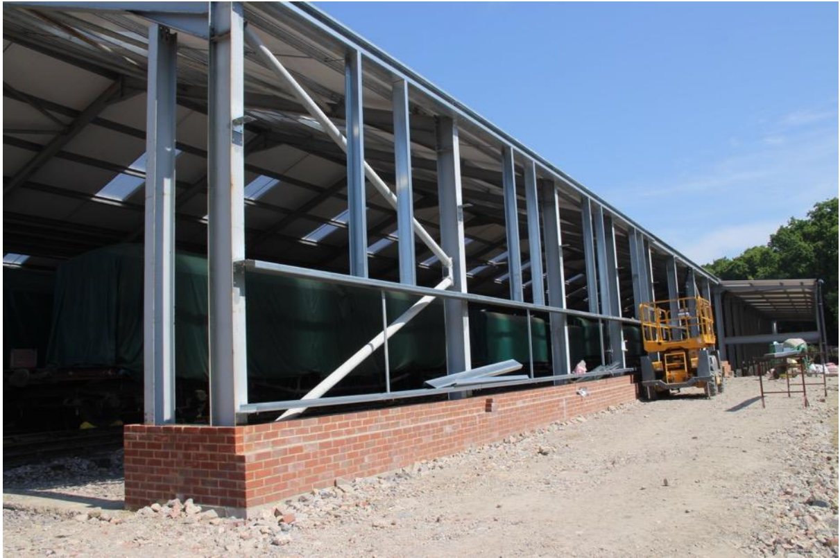
On the eastern side the cladding rails are also almost complete
