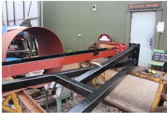
Gantry Under Overhaul
