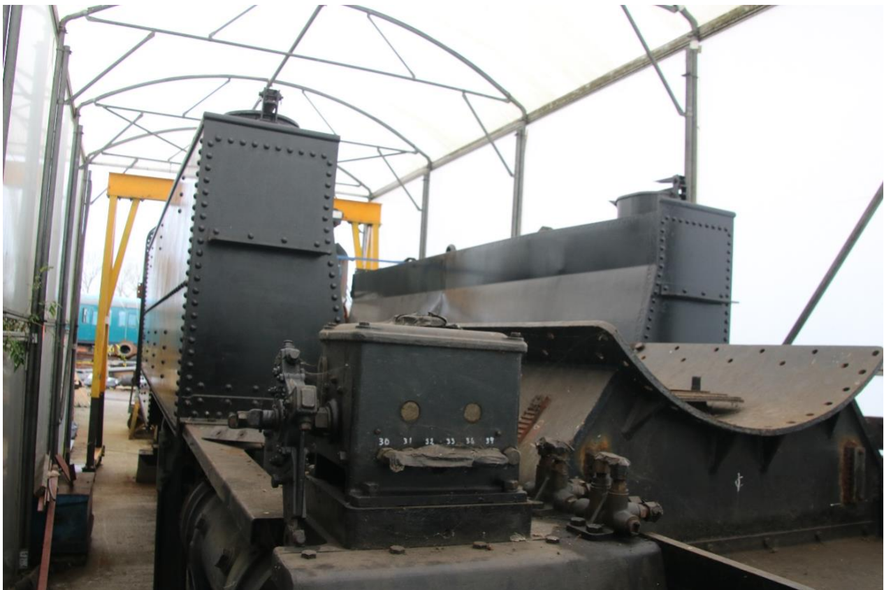
Side Tanks in their final position
