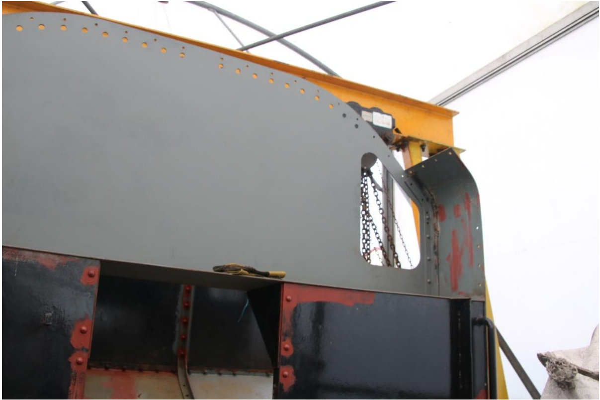
Cab Side of the Bunker showing the shelf which the Tool Box sits on
