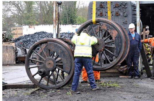
Two wheel sets being set down in the yard.
