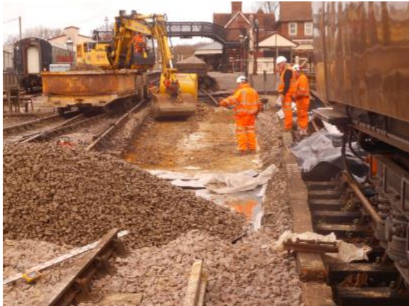
Scraping out the ballast and mud.
