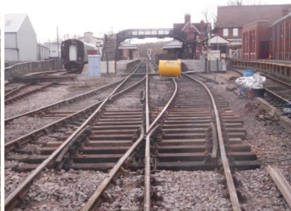
All connected by the end of day three.
