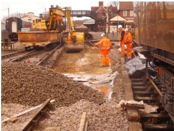
Scraping out the ballast and mud.
