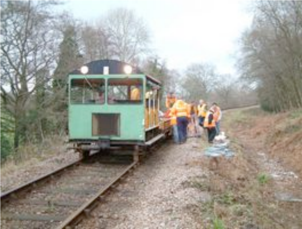
Picking up the fencing gang – 16 Jan 2011.
