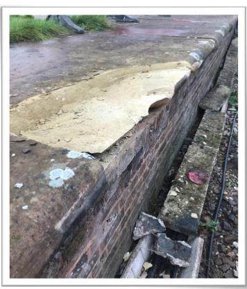
One advantage of the complete replacement is that many of the old stones are still in serviceable condition and can be re-used now or in the future for repairs on other platforms.
