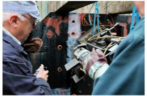
Using A Magnet Base Drill On The Frames
