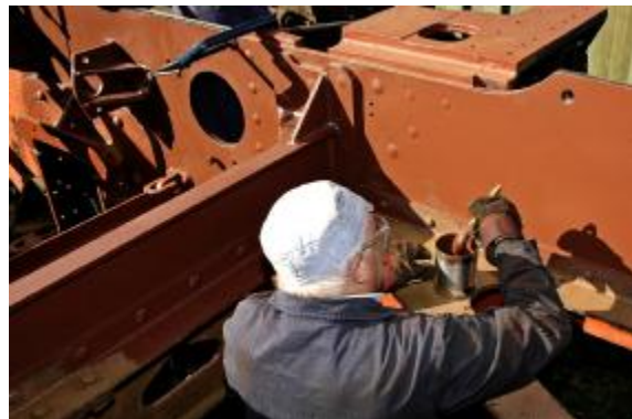
Repainting the frames after needle-gunning.
