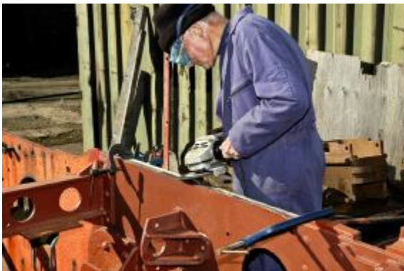
Dressing flame cut frame edges.
