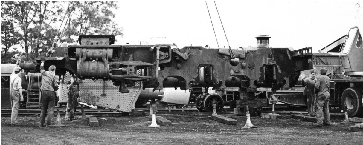
Frames after lifting from the wheel set.
