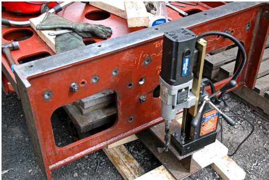
Stretchers bolted in position for drilling
