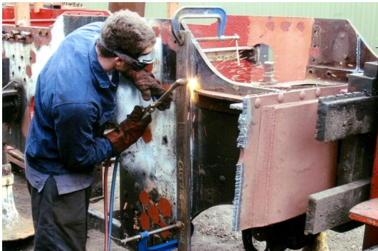
Cutting the hind drag box from 78059
