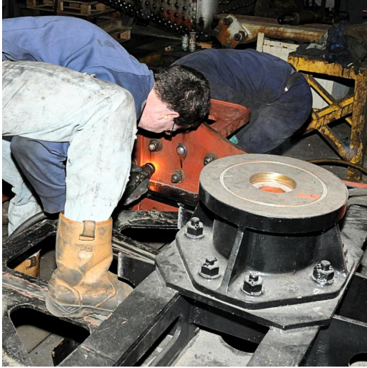
James & Darren closing gusset rivets
