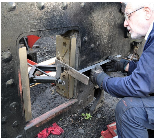
Checking a horn guide liner against a frame button.
