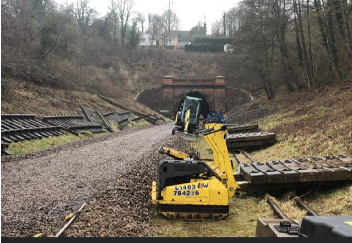
Track removed north of Sharpthorne Tunnel.
