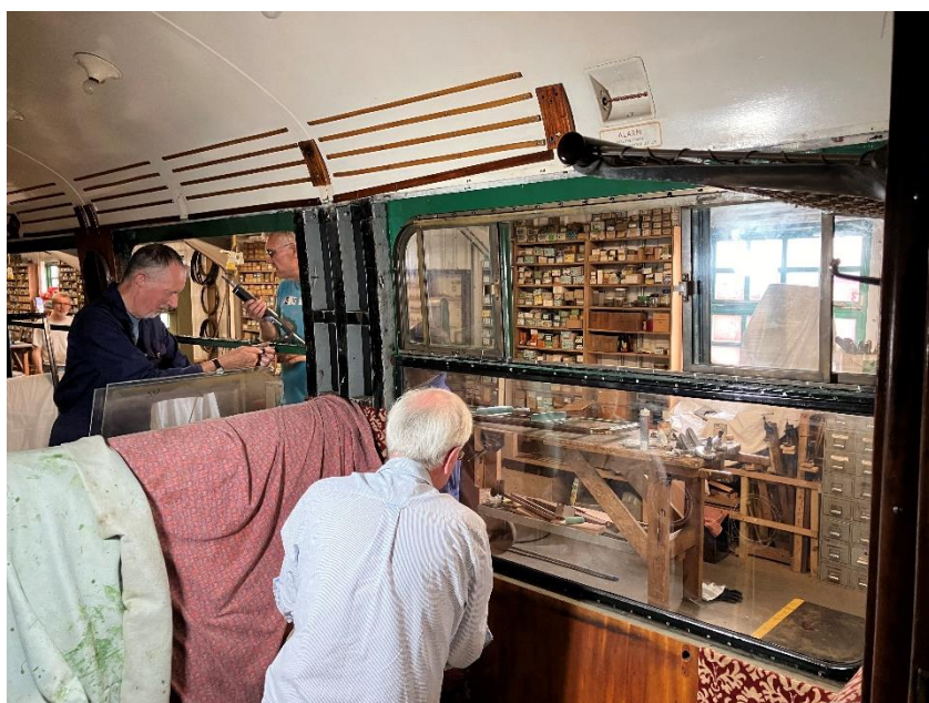
Screwing into place the inner frame for one of 1482's sidelights. July 2024
