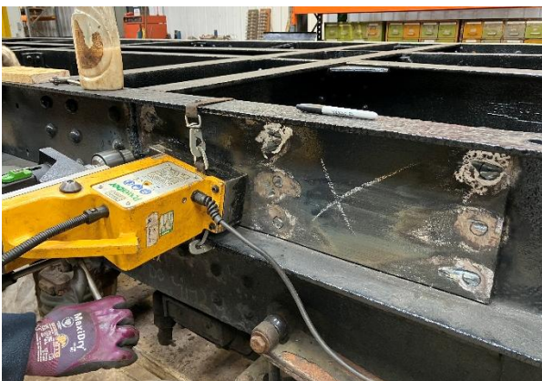
Drilling through rivets on the underframe. 7 Mar 2026
