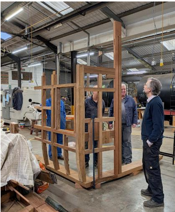
The north east corner being trial assembled on 17 December 2025
