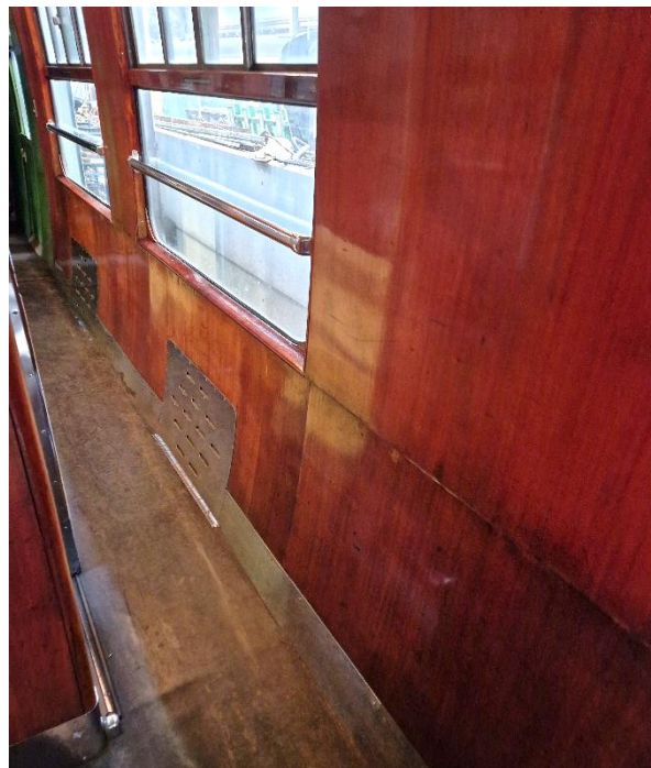
2526's corridor after completing work to the mouldings and kick plates. 11 Mar 2025
