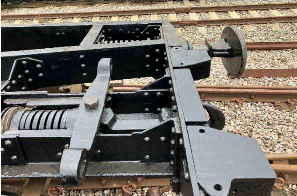
South end buffering and drawgear refurbished and refitted. 4 Nov 2025
