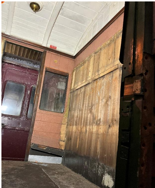
The first compartment to be stripped of its varnished mouldings etc. 4 Mar 2026
